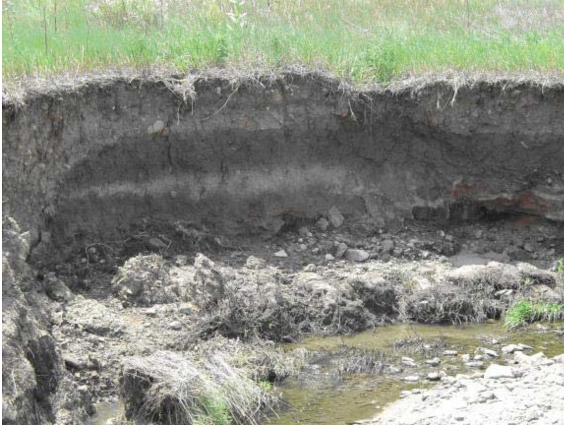
Figure 5-3 Example of Streambank Erosion along Massey Draw, upstream of Chatfield Reservoir
